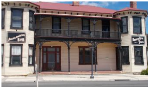
141 Weld St, Beaconsfield
