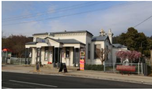
121 Weld St, Beaconsfield
