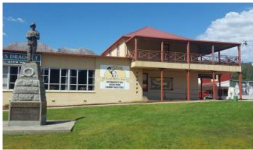
1 Orr Street, Queenstown
