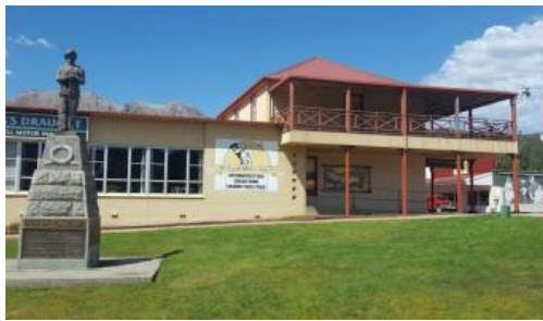
1 Orr Street, Queenstown
